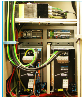
4x transformers 170 kVA MF and 2 inverters MFC-3015w
